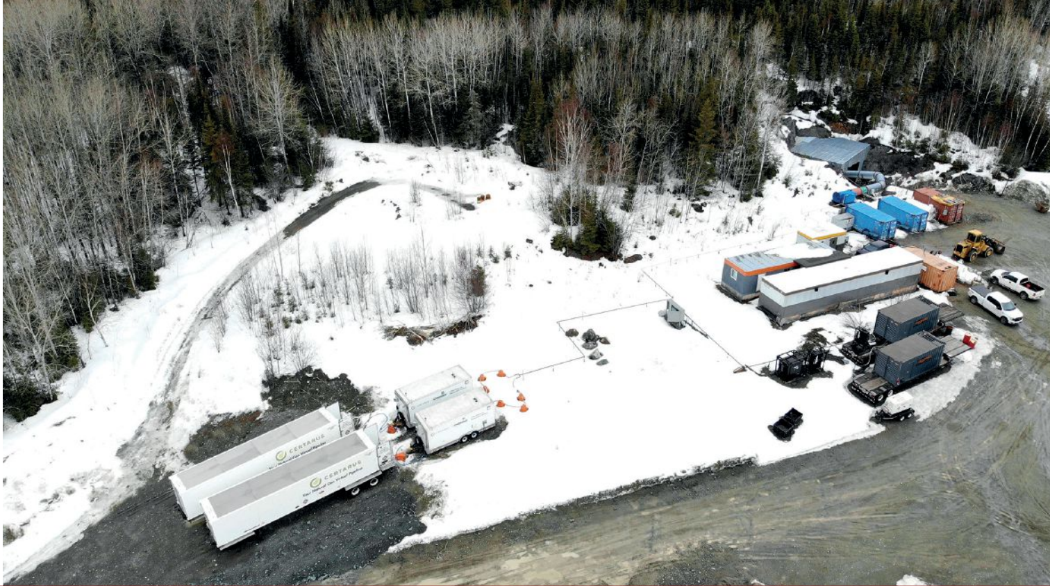
Aggreko's CNG-based virtual power pipeline approach was recently utilized at Labyrinth Resources' gold exploration project on the Quebec-Ontario border. With no grid connection available, the miner needed a portable power solution that would operate in the harsh onsite conditions, while reducing the carbon emissions and high costs associated with diesel. Photo: Aggreko
