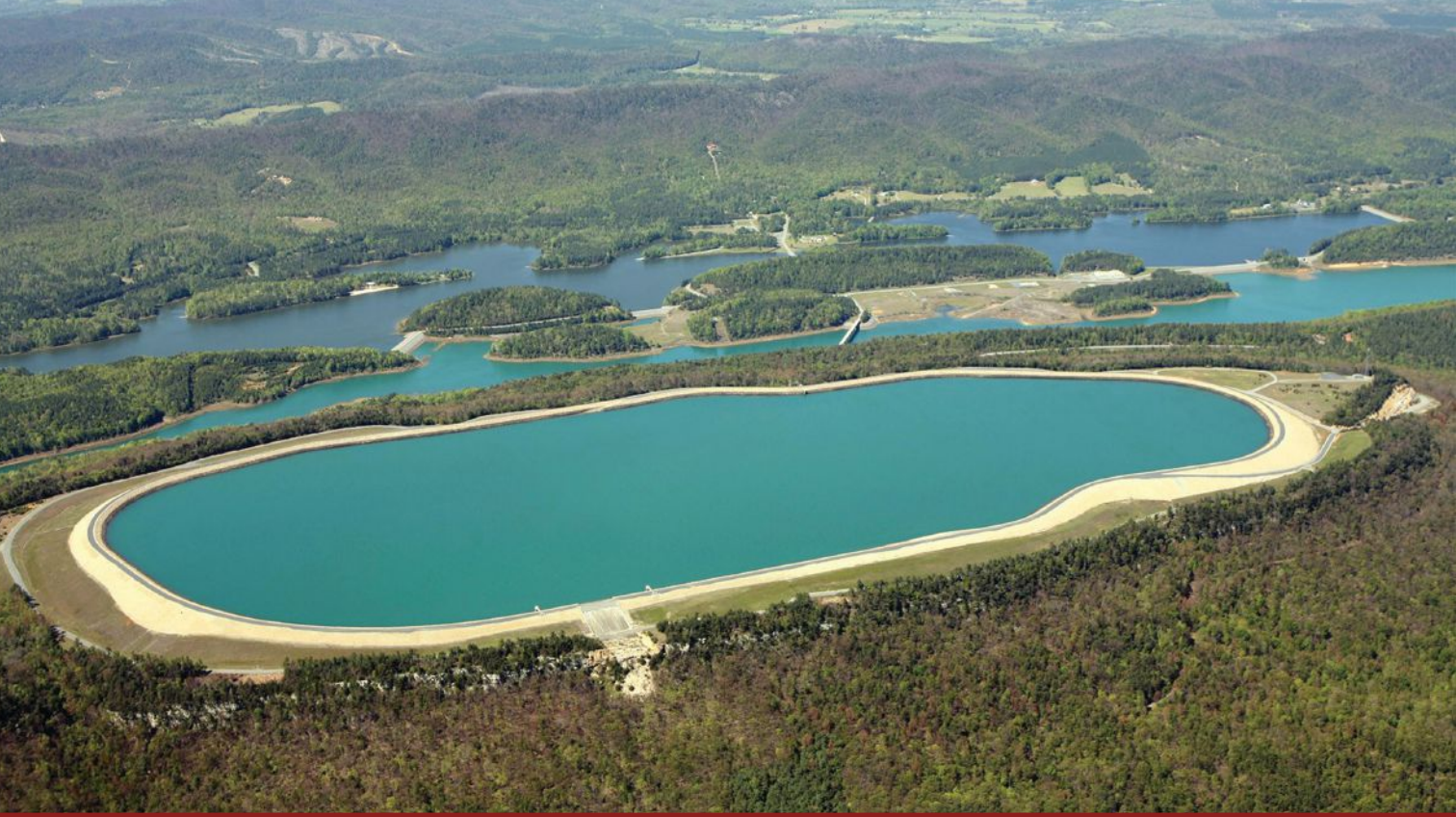
The Rocky Mountain pumped storage facility in Georgia can store nearly 7,000 MW hours to be used when needed. Photo: Stantec
